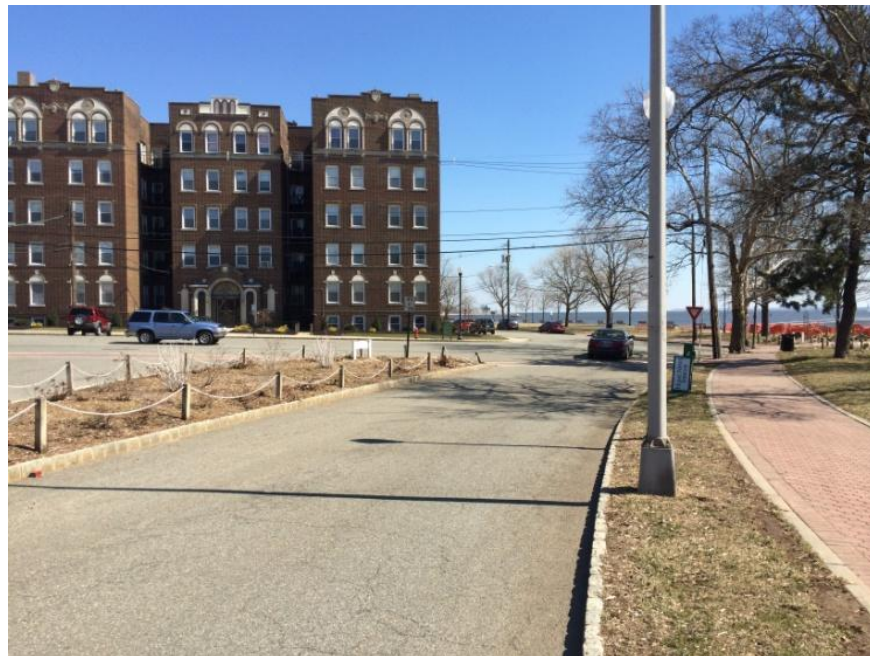
Figure 4: The partially subgrade units of this apartment building at 44 High Street were flooded during Sandy.
