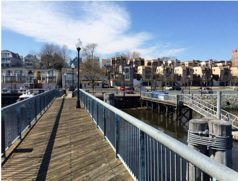
Figure 2: A view taken in February of 2014 from a pier at the Harborside Marina looking back to Front Street. The public marina was hit by a surge that swept over the protective wind wall and swept boats and gangways into the parking lot and street.
